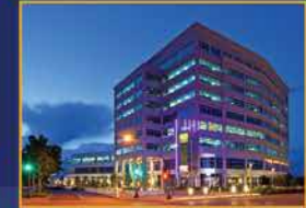
VILLAGE CENTER STATION I
